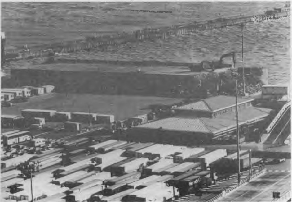
The pens as demolition started and showing the in-filled Camber.
