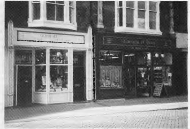
THE RESTORED SHOPS IN CANNON STREET
