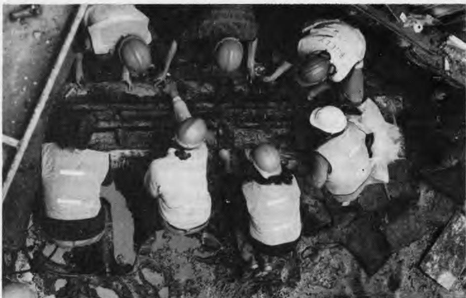
PLATE III: Preparing to lift a cut section of the boat
