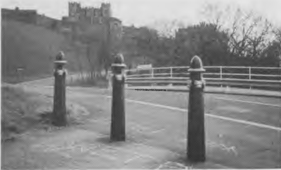
The work completed and Joe Harman's dream comes true
