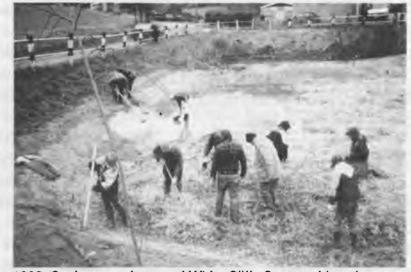
1992 Society members and White Cliffs Countryside volunteers puddling straw and clay to re-line Lydden Pond
