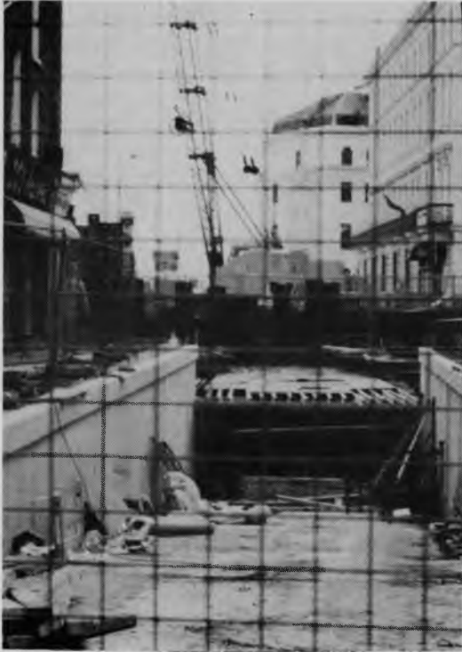
THE SUBWAY AT BENCH STREET UNDER CONSTRUCTION
