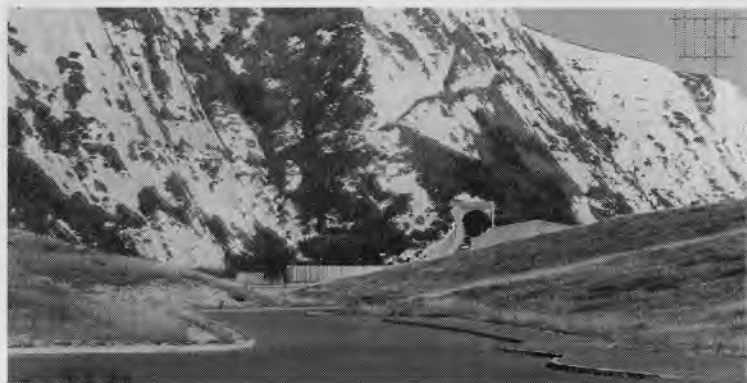
The access tunnel opening on to Samphire Hoe.
