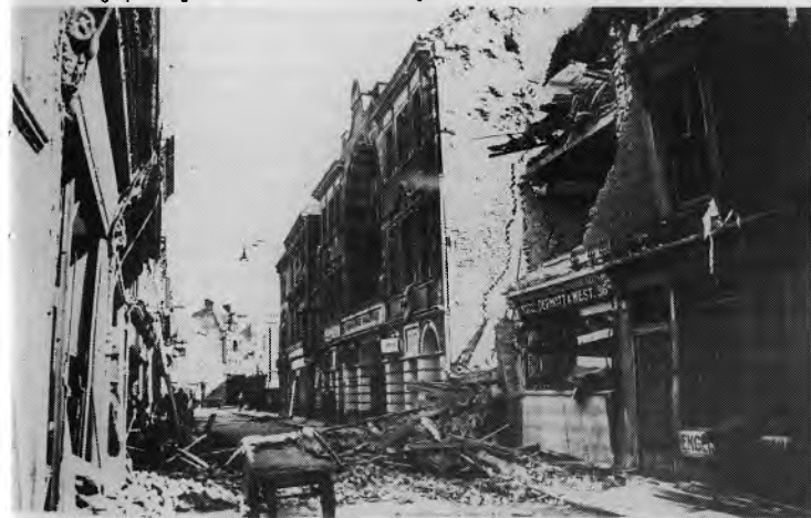
THE DAMAGED 'ROYAL HIPPODROME' and adjacent buildings, looking up Snargate Street towards New Bridge
