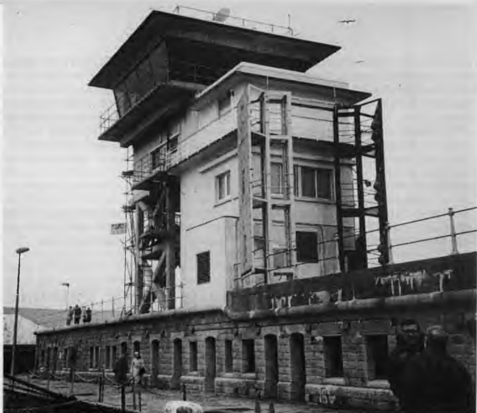
THE CONTROL BUILDING AT THE END (ALMOST) OF THE EASTERN ARM
