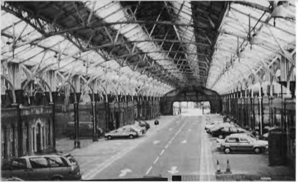
THE SPACIOUS PARKING AREA AT THE CRUISE TERMINAL
