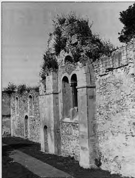
The north internal wall of Old St James's church.
