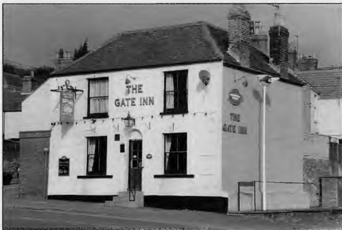
The Gate Inn, which stands slightly townwards from the site of the original turnpike gate.
