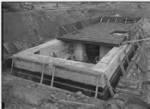
Magazine under construction at Capel Battery
