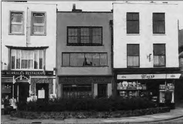
An exterior view. 1960
