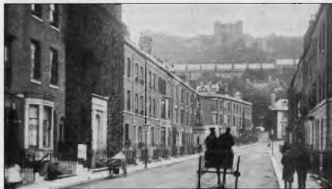
Castle Street in 1914. 'Riverside House' at left covered with a red-leaved creeper.
