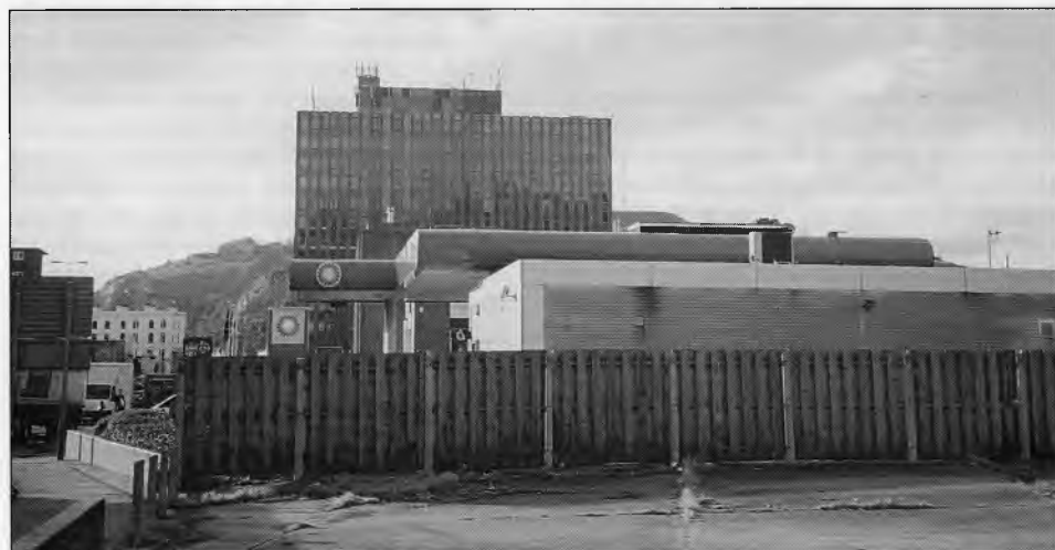
Dover's infamous eyesore - Burlington House seen over the BP garage and adjacent derelict site
