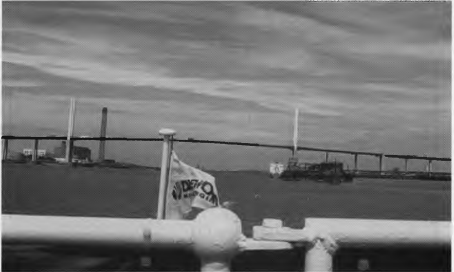
Queen Elizabeth II Bridge - Dartford River Crossing
