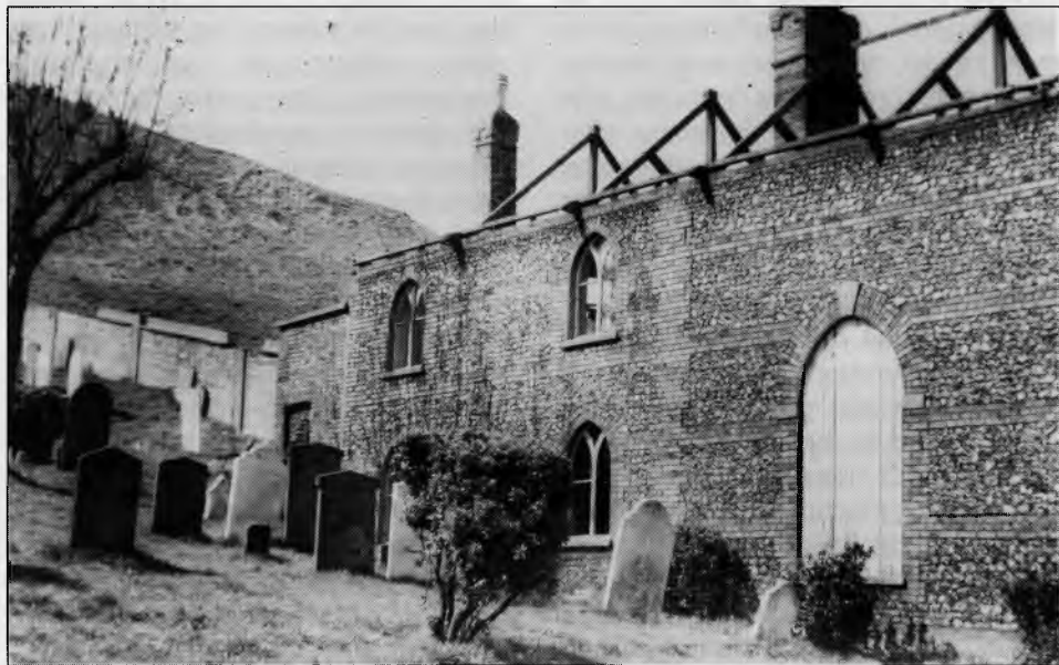
Caretaker's cottage without roof
