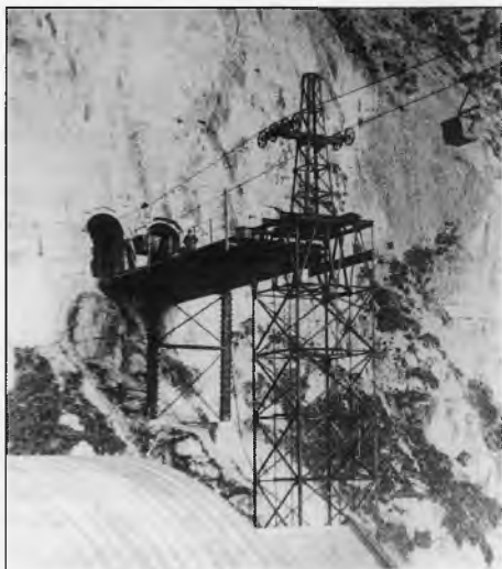
Aerial ropeway emerges through the cliffs on the Eastern Arm
