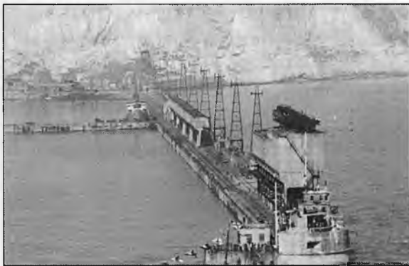
Eastern Arm with its aerial ropeway and coal staithe
