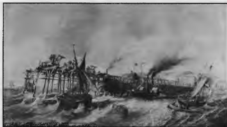
Stanfield's painting of the building of the Admiralty Pier
