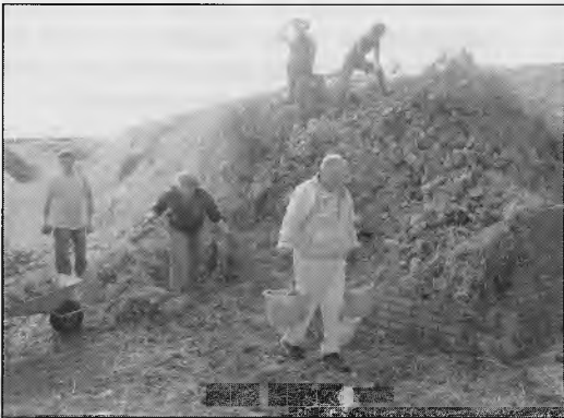
Working progress at the Drop Redoubt
