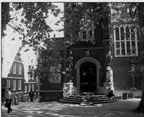
Hall entrance and lane
