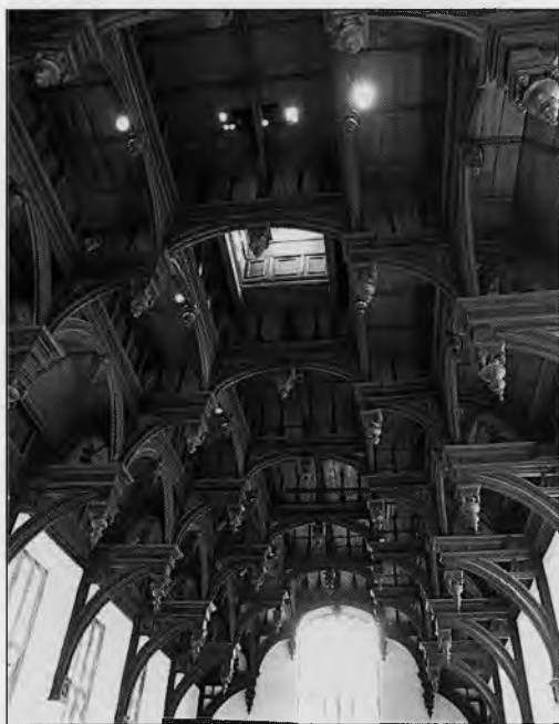
Double hammer beam roof, dining hall, Middle Temple Photo by J. Pople
