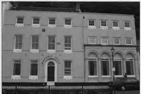
Dover Masonic Hall
