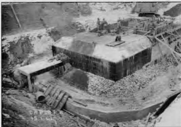
Capel Battery Underground Construction
