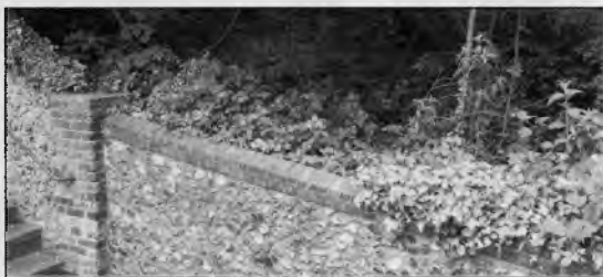
Effingham Steps after final clearance
