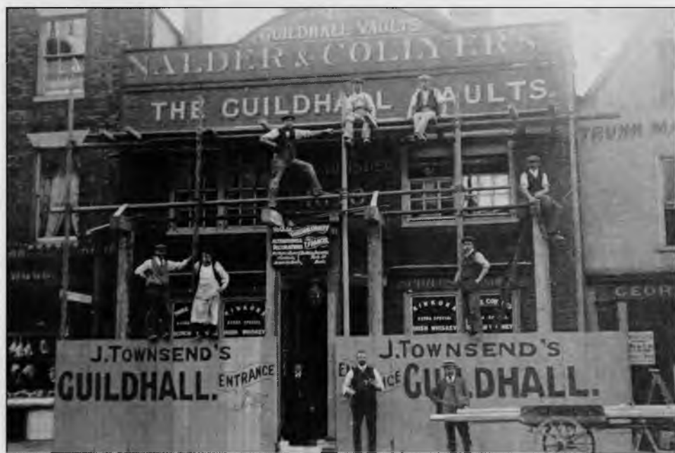
Renovation of the Guildhall Vaults © James Ferrissey
