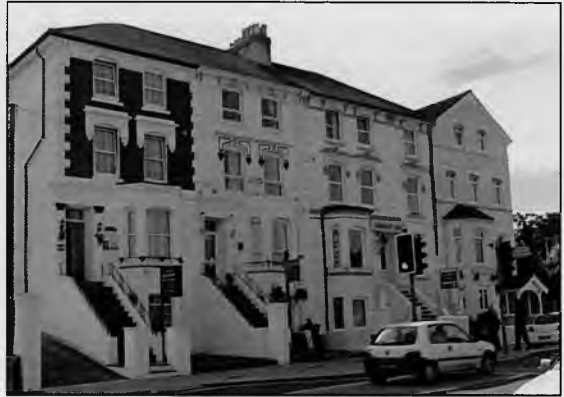
Completed properties opposite Dover Priory station
