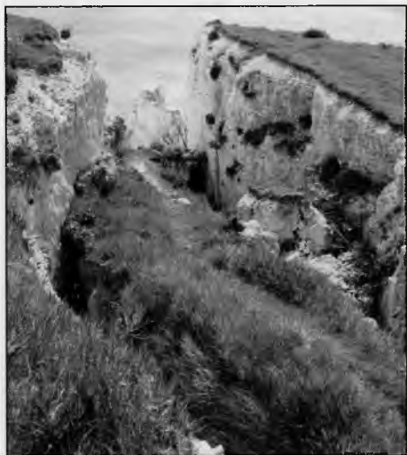
The White Cliffs showing erosion
