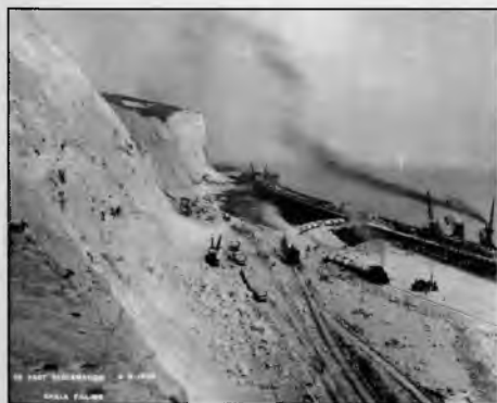
Eastern Arm Reclamation April 1900 © DHB Archives
