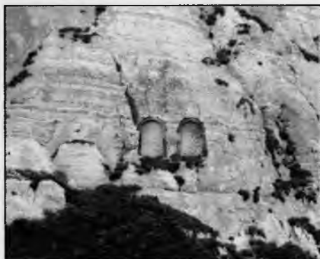
Eastern Docks - Aerial Ropeway Tunnels - LS 2010
