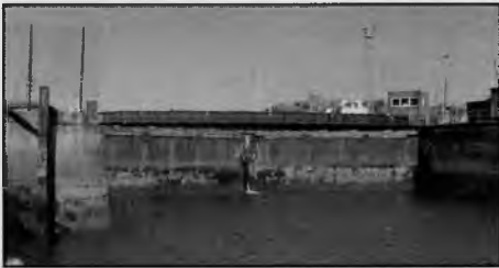
Present Mitre Lock Gates to Wellington Dock that Retain Water within the Dock when Sea Levels are low but cannot prevent water flowing in when sea levels are high © Alan Sencicle 2009
