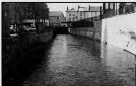
Dour in Full Flood Looking Towards Park Street February 2014 © Lorraine Sencicle
