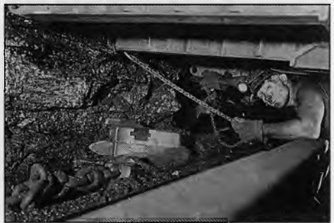
1980 Setting Steel Bars
