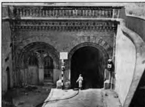
Western Heights North Entrance Tunnel 2016
