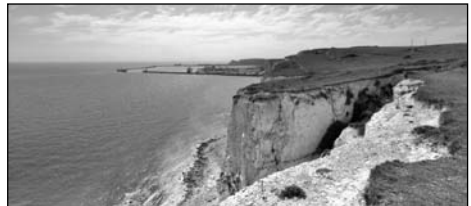
Damage to the Cliffs East of Dover
