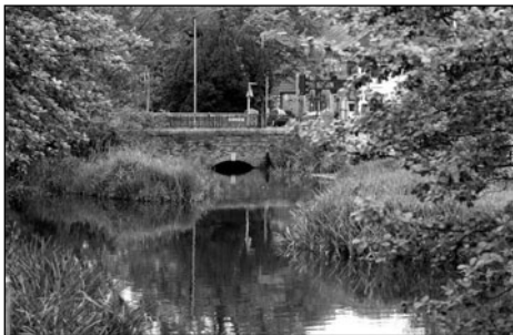
River Dour Bridge Near The Red Lion Pub
